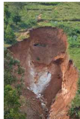
Figure 6—Tunnel into highwall (Rupprecht, 2015b)
